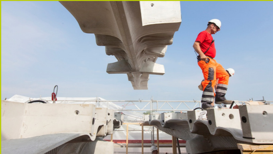
Figure 10: Photograph of the Implementation of the concrete Smart Slabs (Digital Building Technologies, ETH Zürich. Image: Tom Mundy, 2018)
