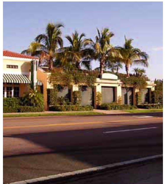
Coconut for dessert? Get it from the roof. Green roof innovation at a restaurant enhances value and enjoyment.
